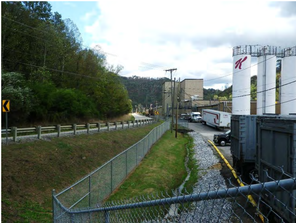
Figure 34. Kellogg plant along KY 194, facing southeast.
