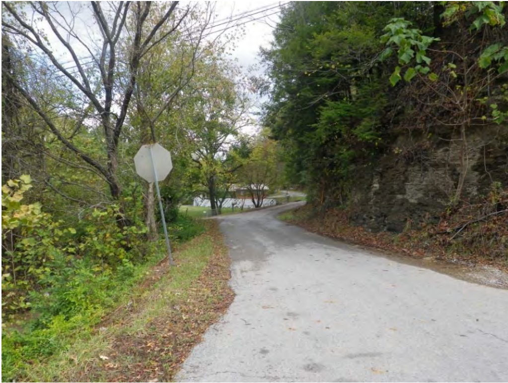
Figure 23. View of Bevins Branch Road, facing east.
