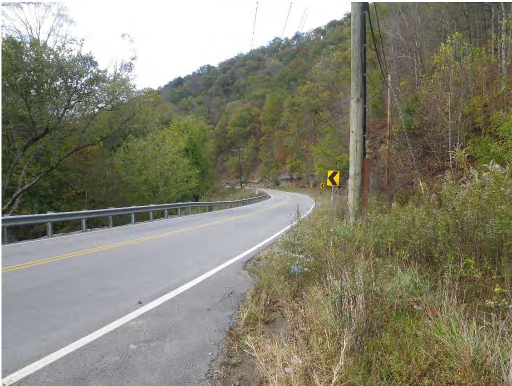
Figure 30. Entrance to Alma Land Waste Area 2A, facing northwest down KY 194.
