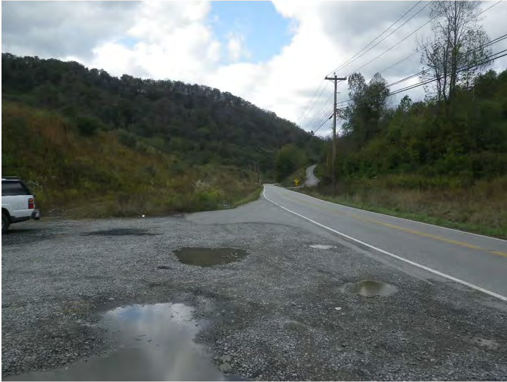
Figure 29. Extended ROW area, facing west.
