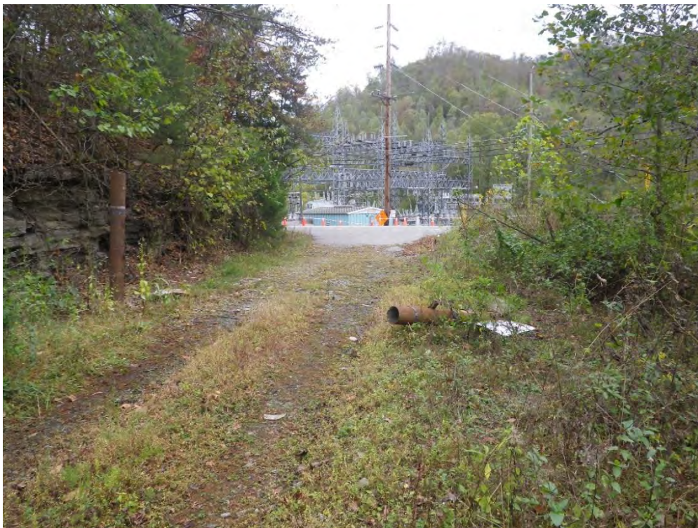
Figure 36. Location of the extension of the ROW and installation of a drainage pipe, facing southwest.
