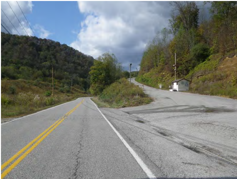
Figure 26. KY 194 near the entrance to Larry Childers Appalachian Land Company, facing west.
