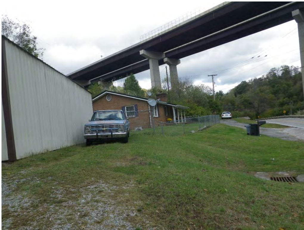
Figure 18. Residential home within ROW at KY 194 and Otis Hollow Road intersection, Parcel 14, facing east.
